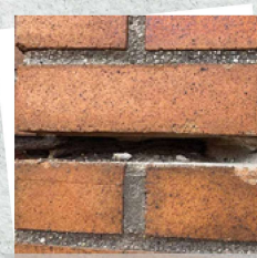
Brick & Mortar Joints
