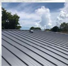
Metal Roofing / Awning
